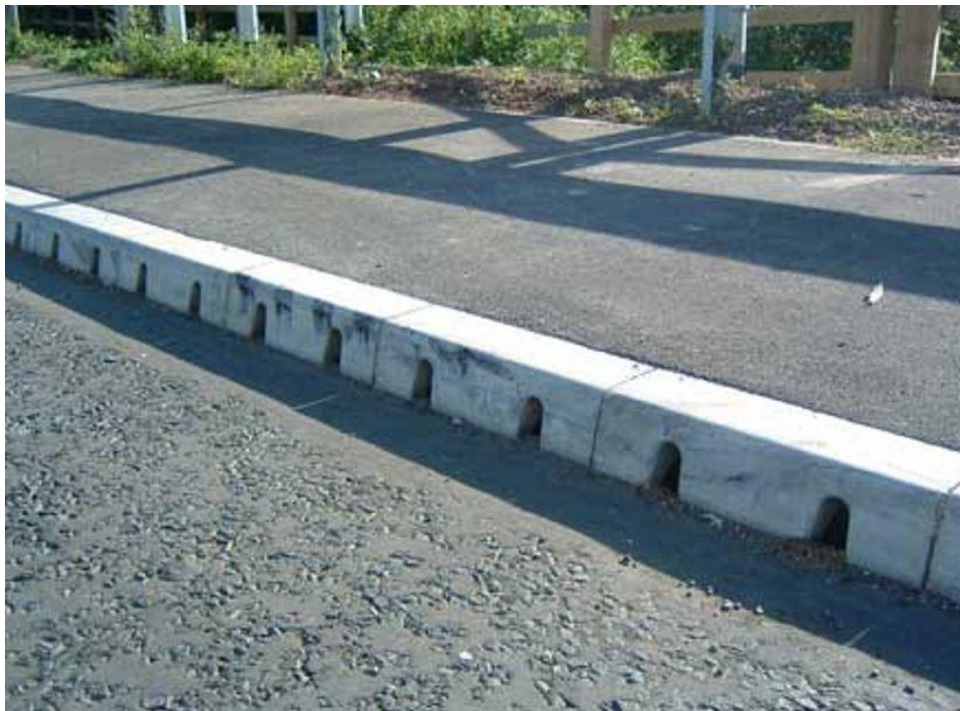
Figure 53: Example of a combined kerb and drainage system
